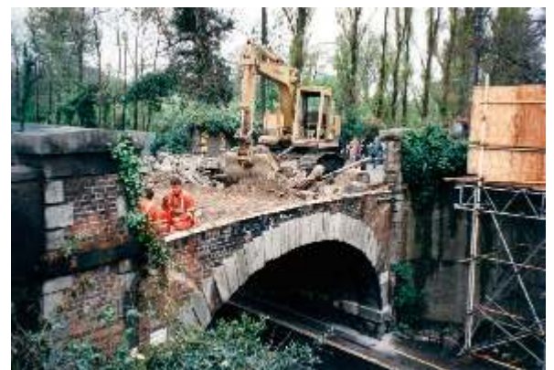
The old arched bridge (seen above) did not offer sufficient clearance to allow installation of the overhead cables for the DART system.
