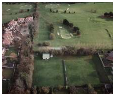
Aerial view of the Grove Tennis Club off Grove Road with the old golf course in the background
